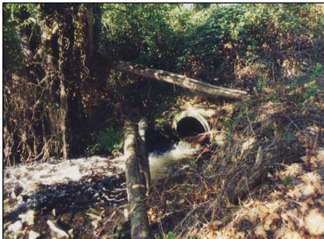
Shoreline discharge outfall.
