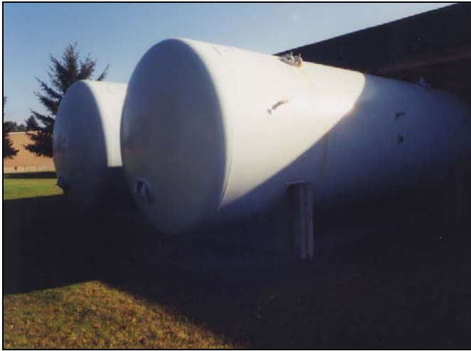
Pressure filtration system.
