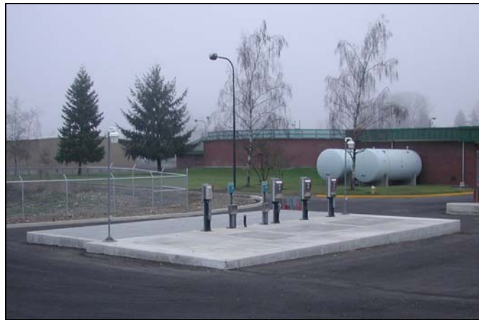
New influent pump station.
