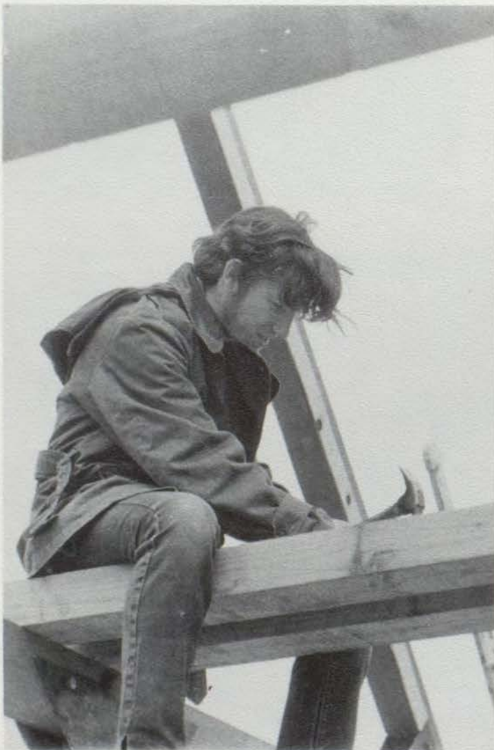
Garry Standley hammers on the main supporting beam.
