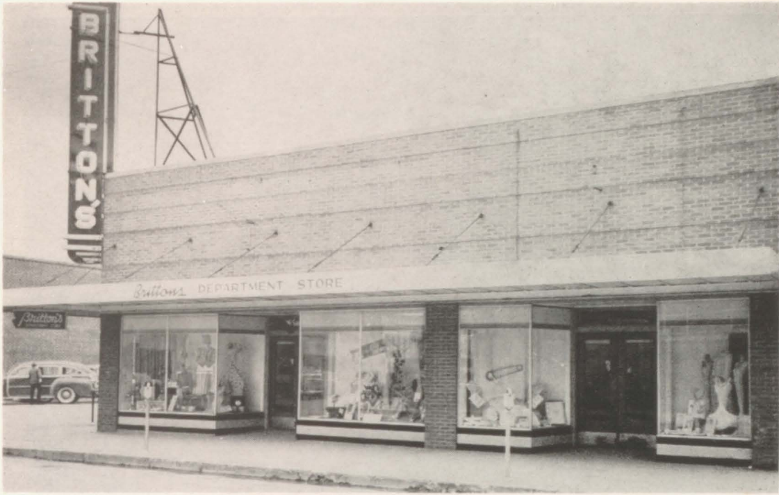
LEBANON'S HOME-OWNED DEPARTMENT STORE
