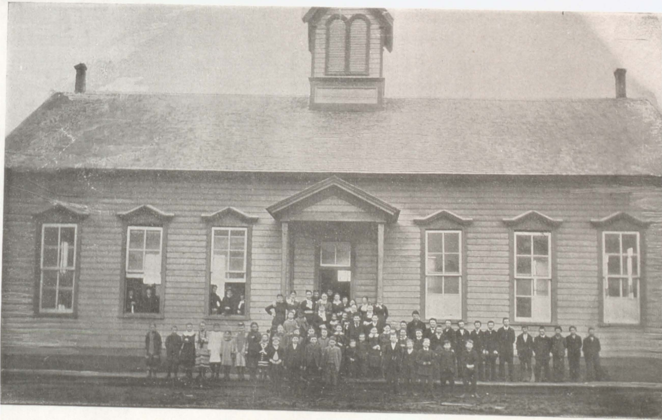
FIRST SCHOOL BUILDING IN LEBANON
